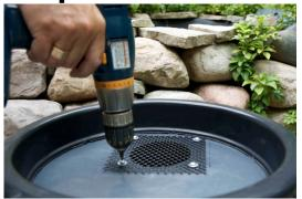
Use drill to fasten screen over hole. Place washers on top of screen as shown above
