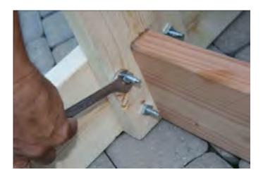
Take the two horizontal and vertical legs and line the holes up and slide the threaded bolts through as shown above. Tighten square nuts onto bolts with wrench and repeat. When you are done you should have the frame assembled and it should look like the picture on the right.
